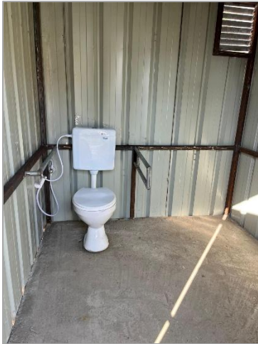
Figure4 Temporary inclusive latrines constructed using locally sourced materials - Humanity & Inclusion, June 2025.
